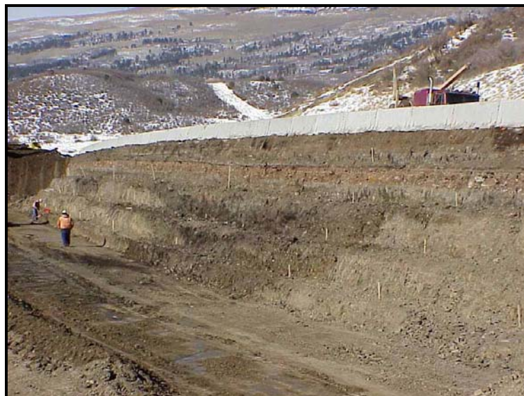
Figure 5. Outline of failure plane during excavation and mitigation of Landslide 1.
