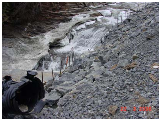
Figure 13. Toe of stone filled slope secured with grouted dowels
