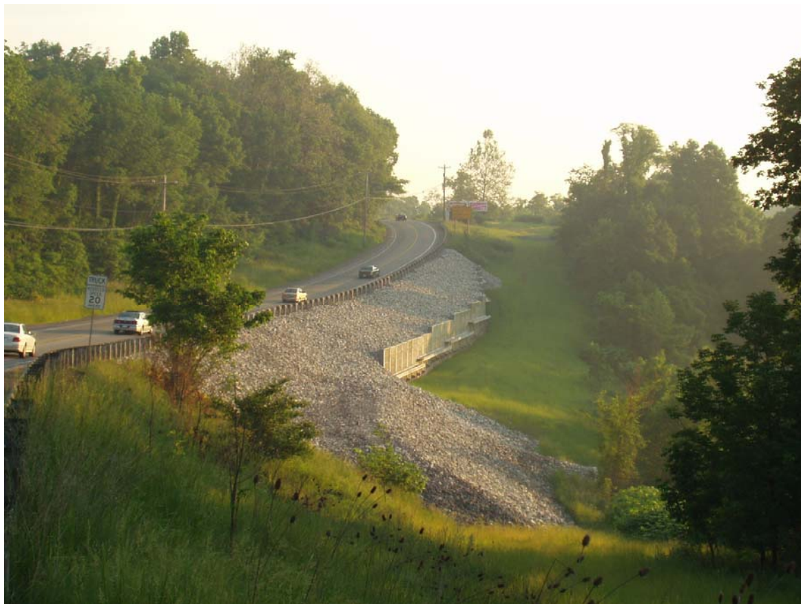
Photograph 3 – Repaired SR 48 Landslide (Northern Retaining Wall and Southern Rock Buttress) Constructed Within the Limits of the Irregularly Shaped Available Existing Right-of-Way
