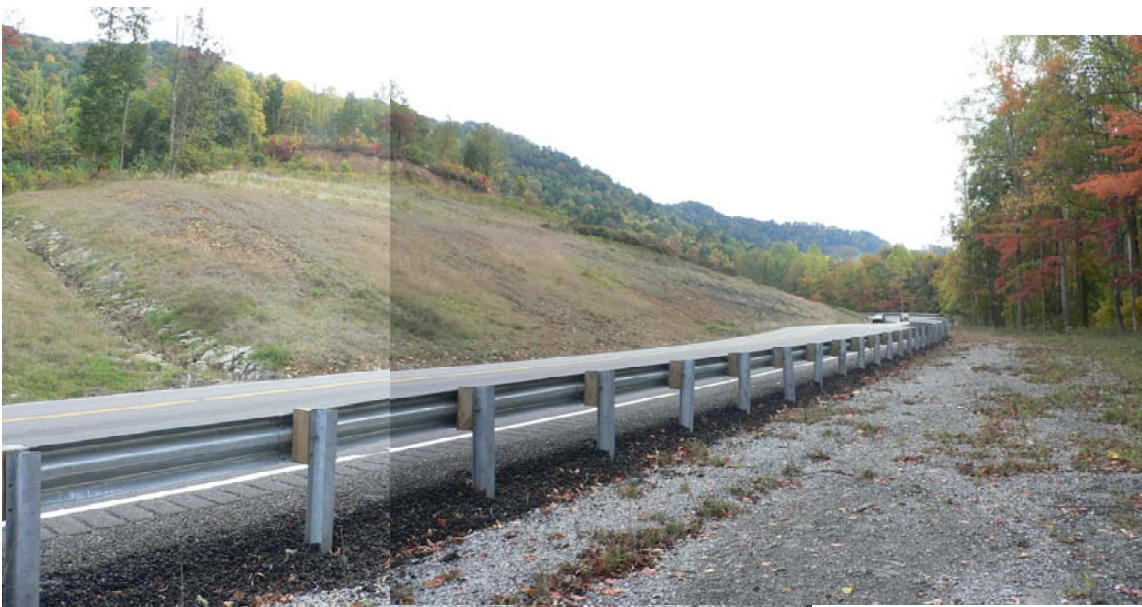
Figure 22. Completed cut slope in colluvial deposits.
