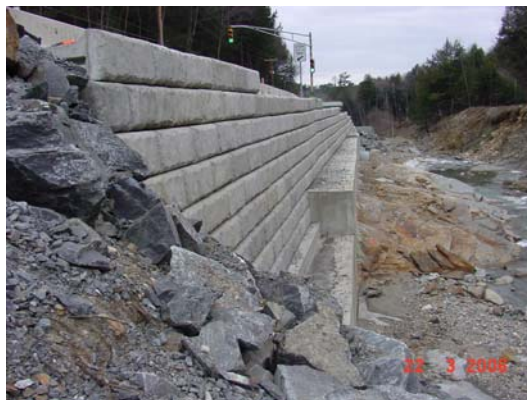
Figure 14. Redi-Rock™ concrete block retaining wall
