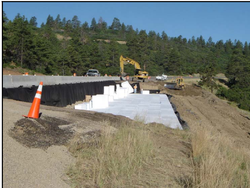
Figure 20. EPS placement in Landside #3 (Replacing Sawdust Fill).
