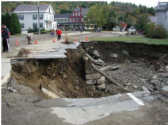
Figure 11. Bridge wing walls damaged and abutment settled 9 inches
