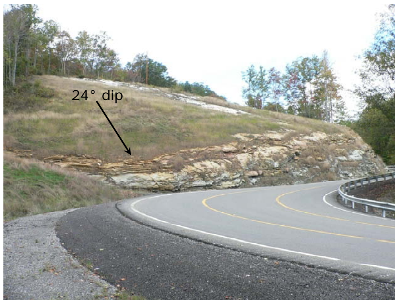
Figure 17. Constructed Cut Slope Involving a Roadway Alignment that is both Parallel and Perpendicular to the Strike of Bedding.
