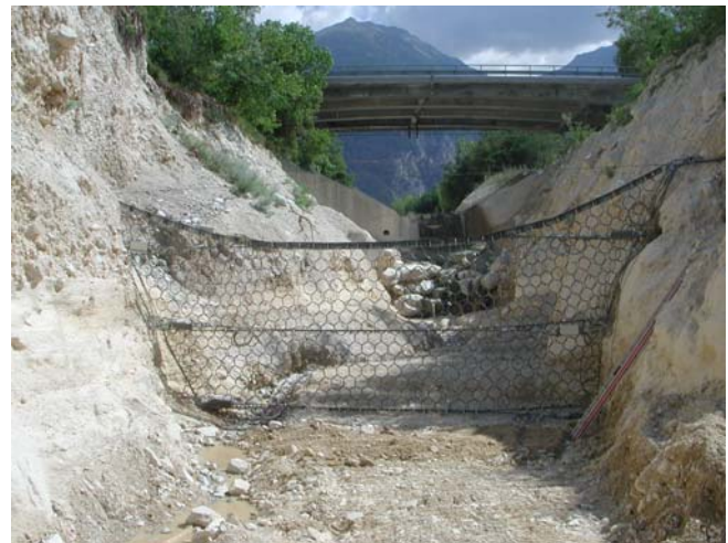
Figure 1. Installed debris flow test barrier.
