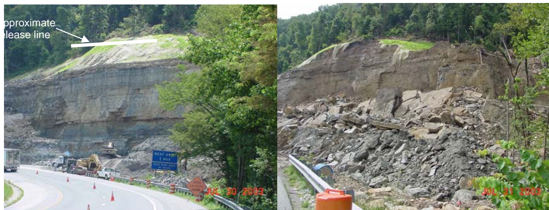
Figure 9. View of the Face before and after large Rockfall, July 30 and 31, 2003
