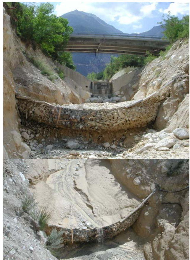
Figure 8. Filled barrier after debris flow event.
