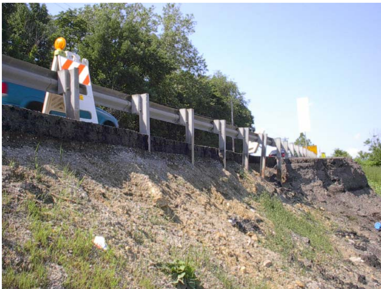
Photograph 2 – Relocated Guide Rails at Head of SR 48 Landslide
