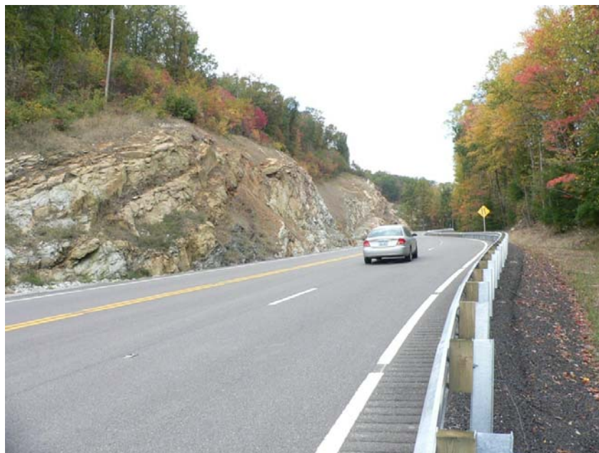
Figure 16. Roadway Centerline Approximately Perpendicular to Strike of Bedding Planes.
