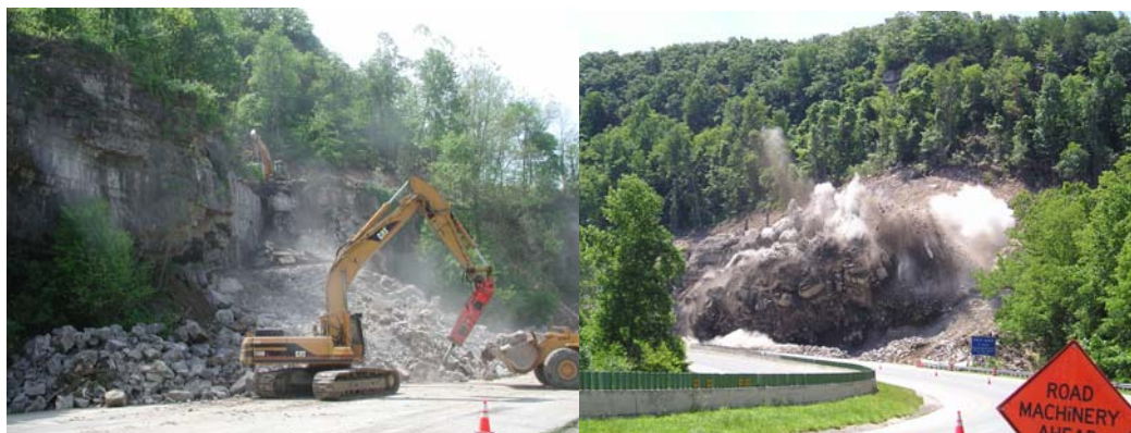
Figure 7. Construction begins, view of blasting and clean-up at the site
