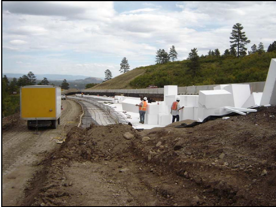
Figure 19. EPS placement in Landside #2.
