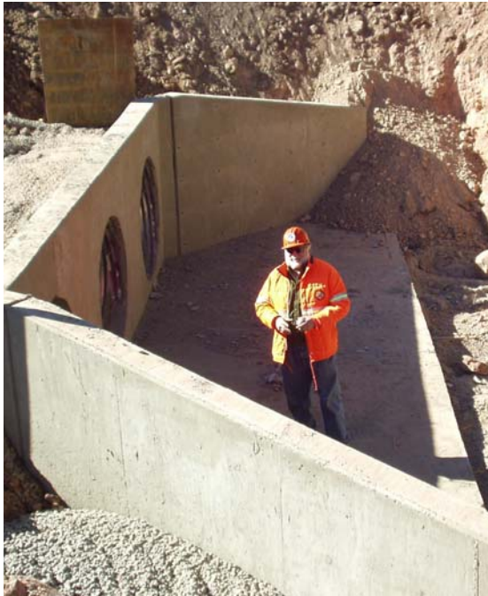
Photograph 4 – Construction view of triple 36 inch culvert inlet on new US 191 alignment near north end of project.
