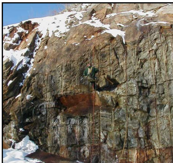
Figure 8 – Wedge of Rock Scaled Before Failure.
