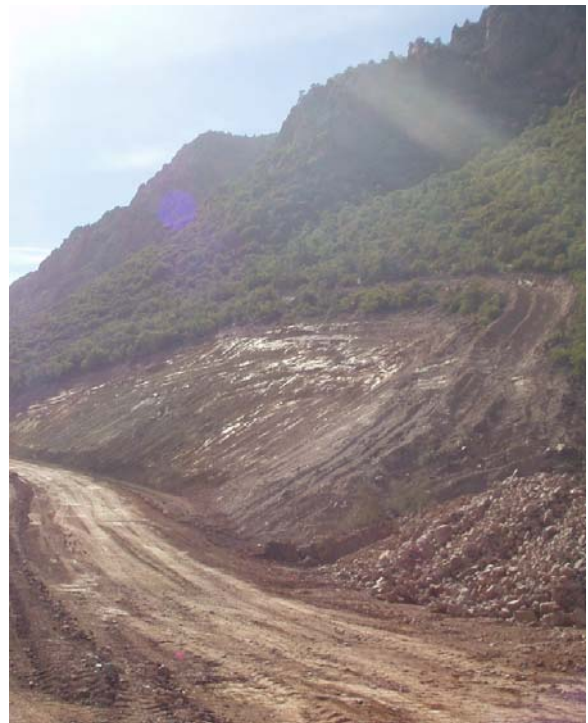
Photograph 9 – Brow or crown ditch installation at south end of new US 191 alignment.
