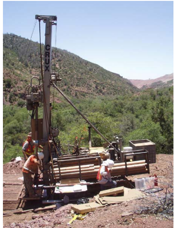
Photograph 6 – Geotechnical Exploratory Drilling along new alignment of US 191 above new Upper Chase Creek Dam.
