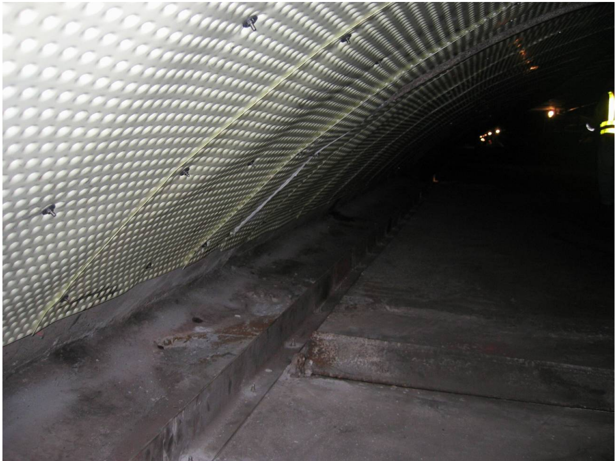
Figure 12. Completed Panning & Drainage Trough
