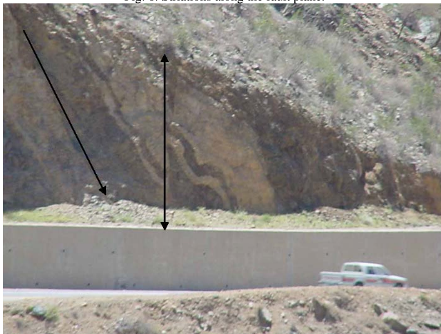
Fig. 7: Folding (single arrow) associated with faulting (double arrow) in the lower part of the descent road, km 22+500-23+000.
