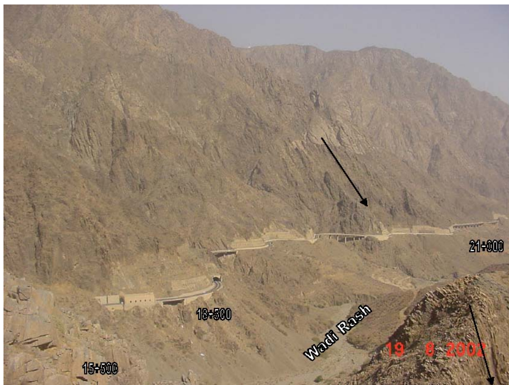
Fig. 3: Westward dipping schistosity dominated along the descent road. Fig. 4: Schistosity (arrows) dipping westward in the western part of the descent.
