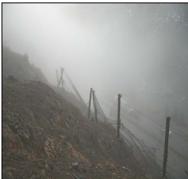
Figure 5: Damage to existing rockfall barrier resulting from April 2004 rockfall incident
