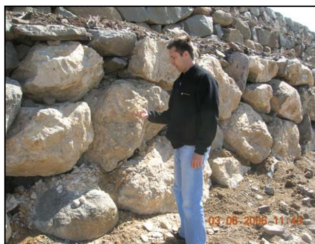
Figure 10: Rockery wall failing because of poor placement of rock and weak unsound rock.
