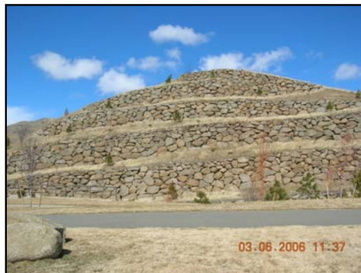
Figure 1: Multitiered rockery wall near Reno, Nevada.
