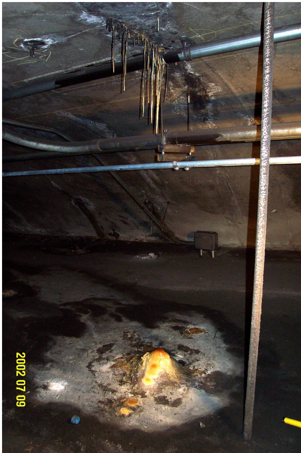
Figure 8. Leakage in Ventilation Plenum
