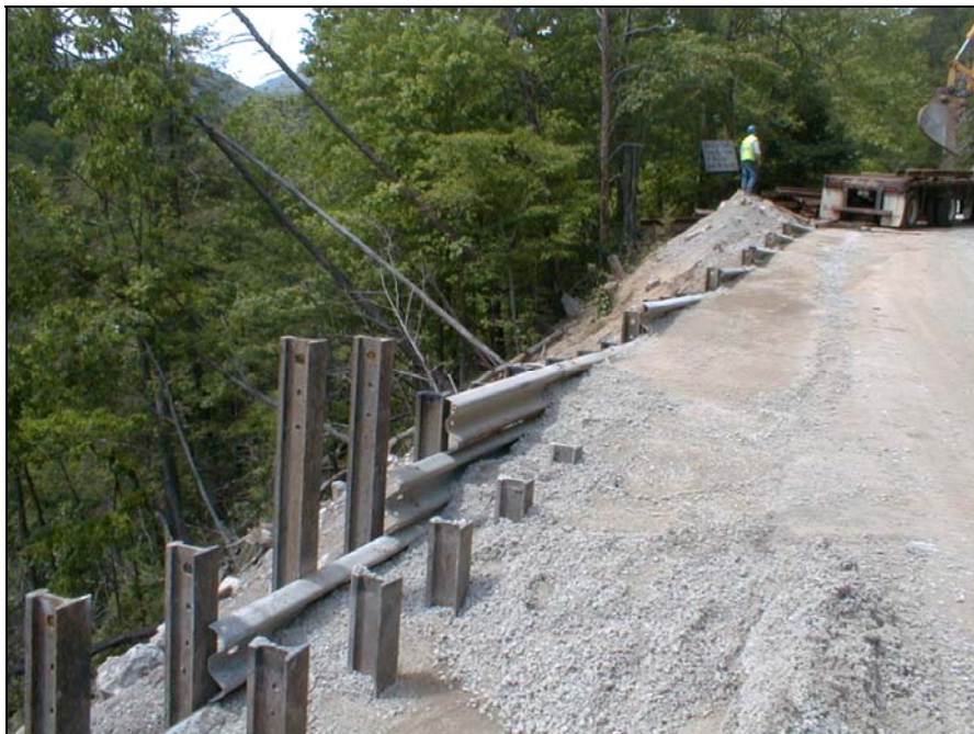
The guardrail was installed in horizontal sections forming small “step-downs” along the top of the retaining wall and shoulder edge.
