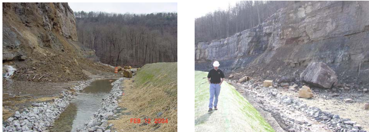
Figure 13. View of Slide Material and Large Boulders Contained in Catchment Ditch
