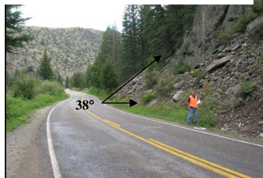
Figure 2: Talus slope with a 38° angle of repose, Taylor River Road, Colorado.
