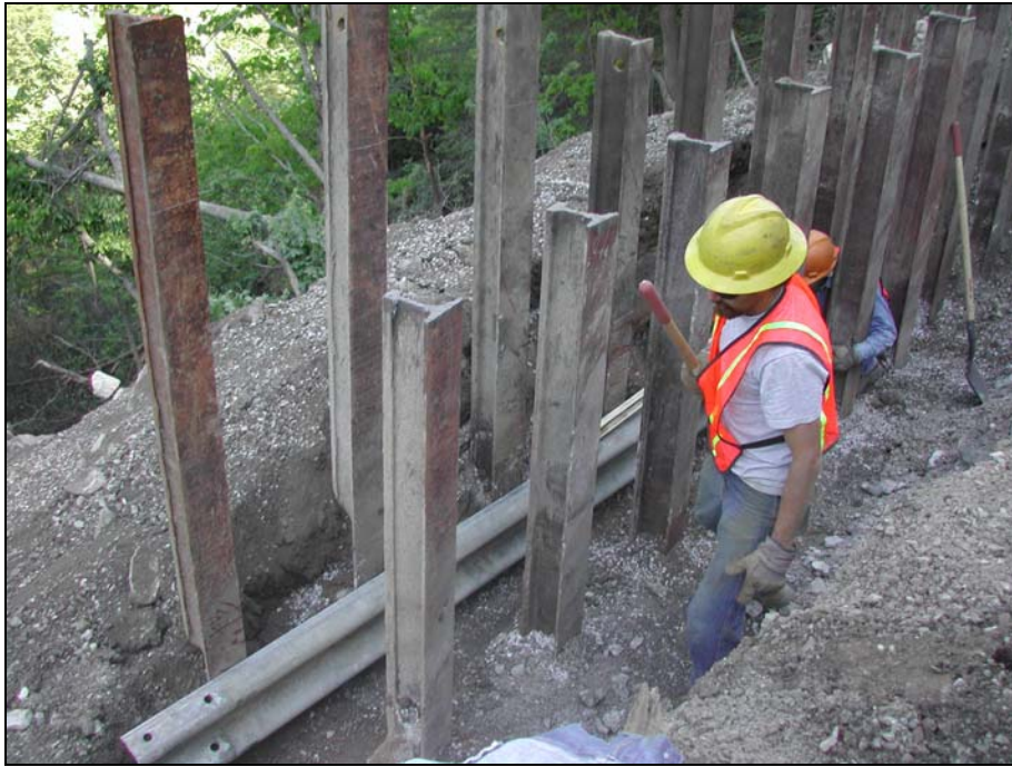
This photo shows the installation of guardrail along the outside row of railroad rails forming the retaining wall to support the stabilized and widened roadway shoulder.
