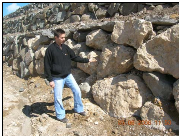
Figure 7: Example of rockery wall failing because of placement and use of weak rock for wall rock.
