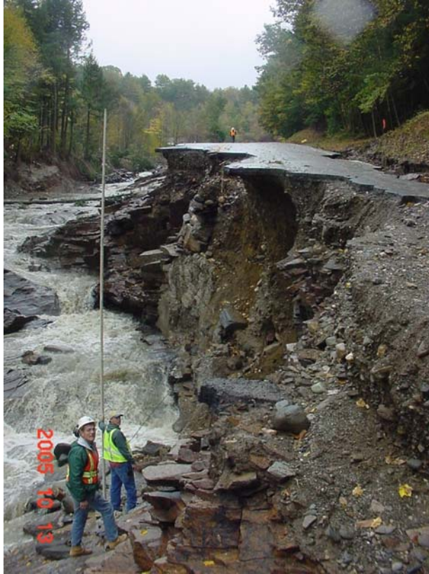
Figure 10. Section of Route 123 stripped to bedrock
