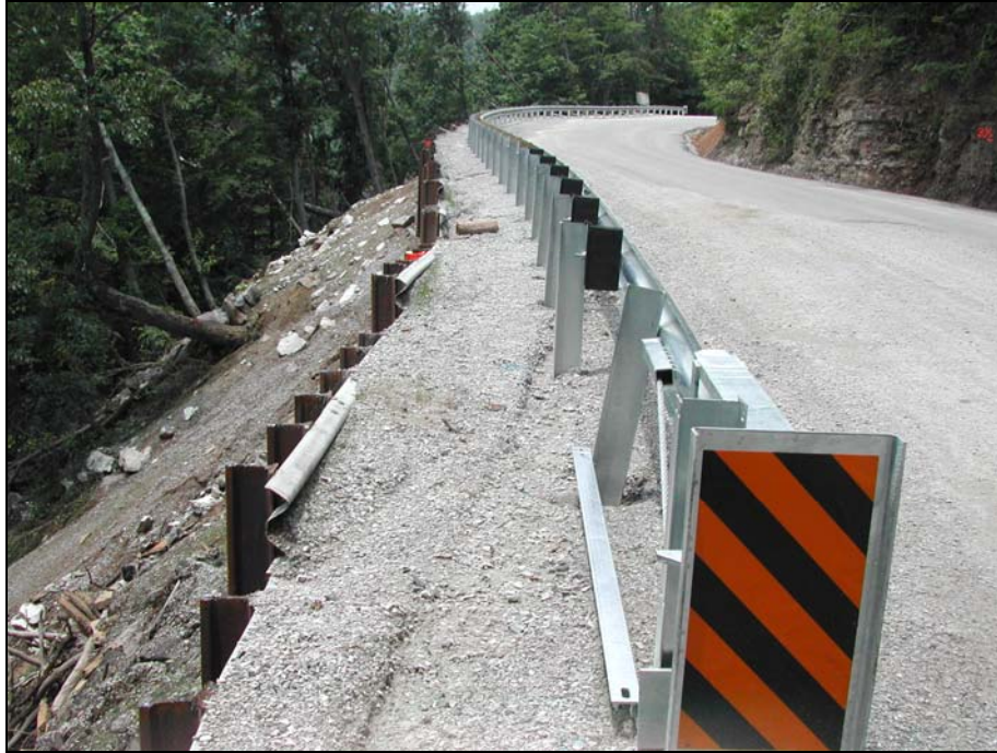
This view shows the completed slide repair site with completed railroad rail wall and newly installed roadway guardrail. The previously undermined section of road was located just to the right of the guardrail near the upper-middle portion of the photo.
