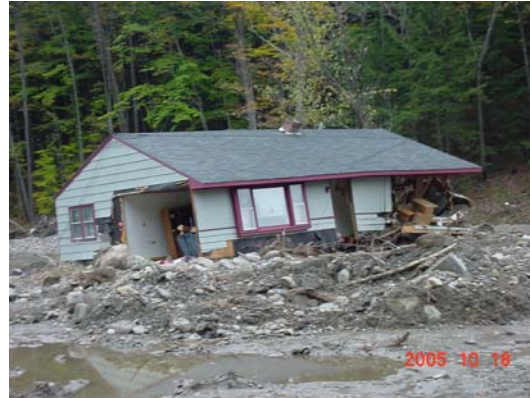
Figure 5. House ripped from foundation
