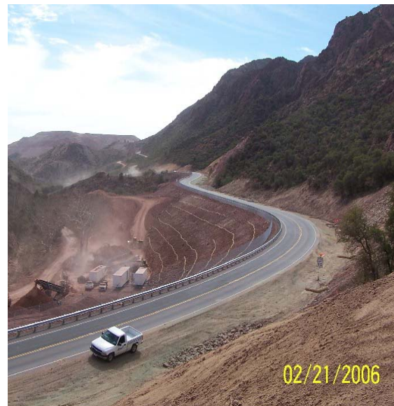
Photograph 7 – Newly constructed alignment of US 191 above new Upper Chase Creek Dam with completed pavement.
