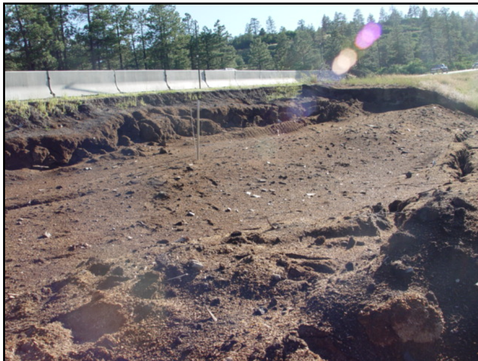
Figure 10 – Landslide 3 - Looking west along US 160 (Foreground is composed of sawdust fill).
