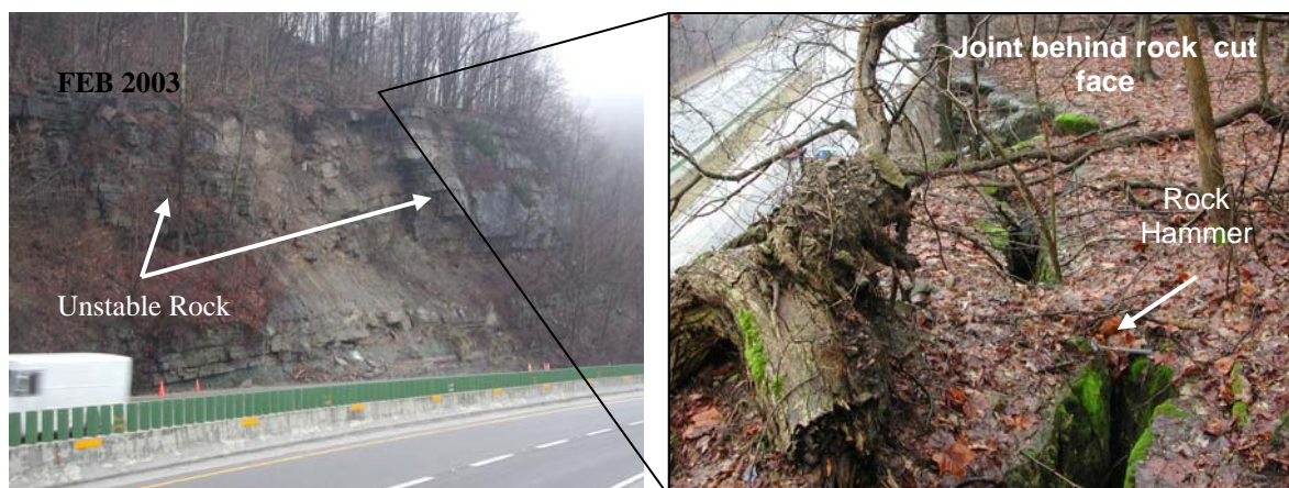
Figure 3. Unstable Face and Joint Behind the Rock face
