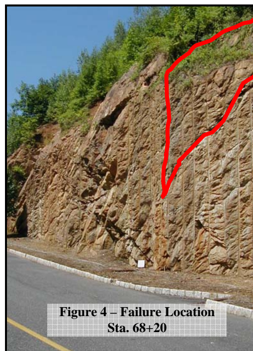
Figure 3 – Failure Surface at Timber Ridge Rd., Sta. 68+20
