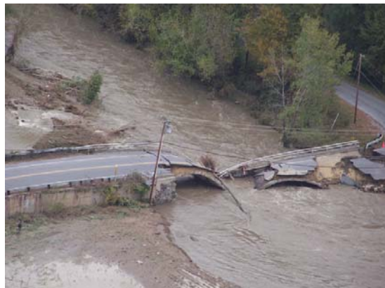
Figure 12. Twin arch bridge washed out
