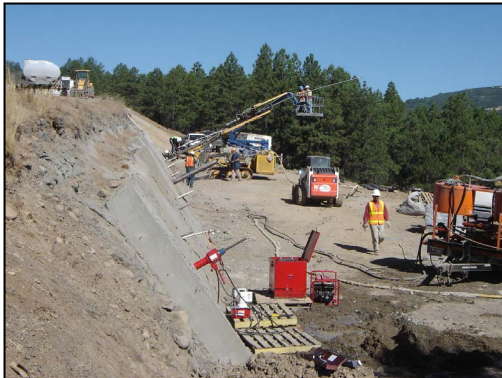
Figure 23. Installation of the Tieback Ground Anchors.
