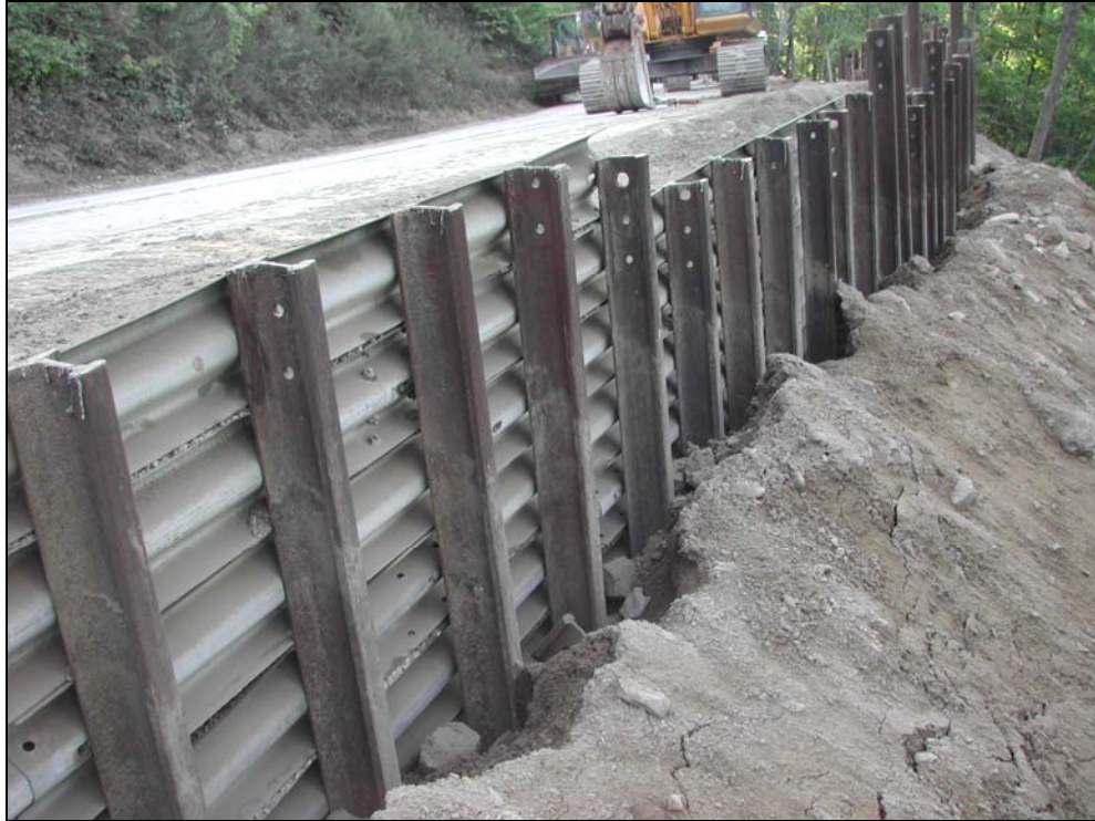
After the guardrail installation and backfill stone placement was completed the RR rails were then trimmed forming the final retaining wall stabilizing the roadway.
