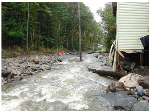
Figure 8. New brook channel cut into roadway
