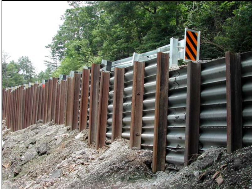
This view of the completed RR rail wall shows the highest portion of the wall at 10 feet (near the middle left of photo). Note the new guardrail installed along the roadway shoulder.
