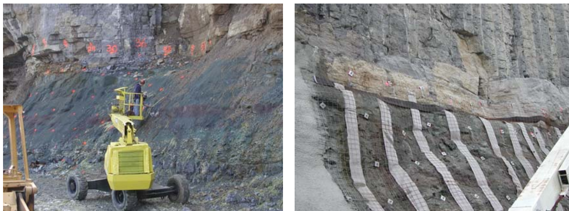
Figure 14. Installation of Shale Cover
