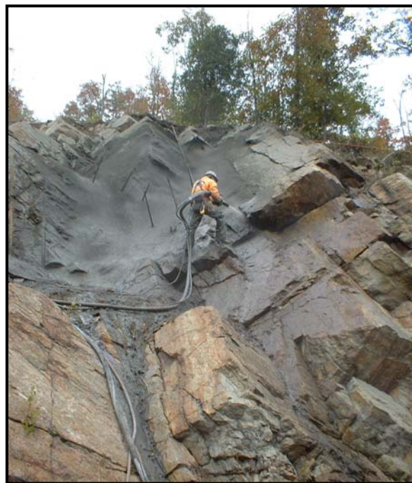
Figure 6 – Bldg. C Overhang Shotcrete Application
