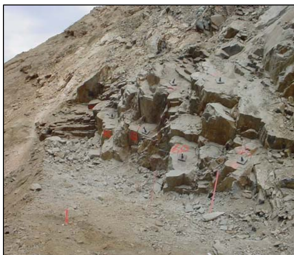
Figure 10 Reinforcement at Overlap
