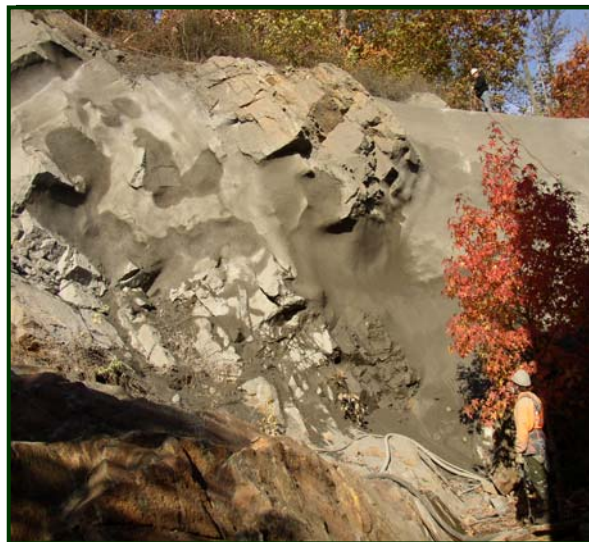
Figure 7 – Final Appearance of Bldg. C Shotcrete Application
