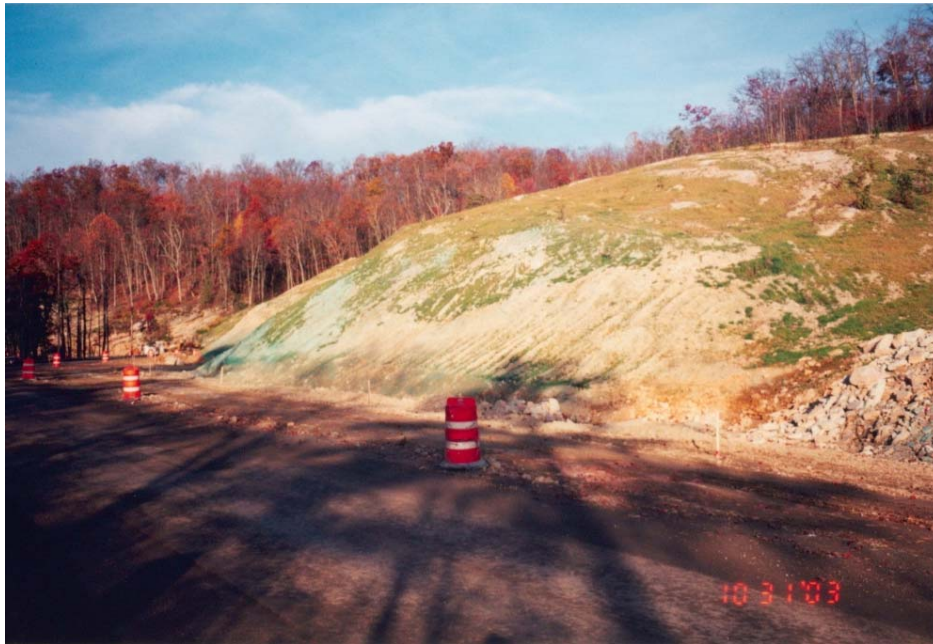
Figure 13. Shot-In-Place Berm
