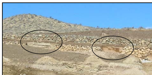
Figure 9: Failure of rockery wall from poor drainage exacerbated by poor rock selection and placement, Reno, Nevada.
