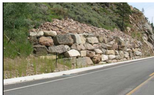
Figure 3: Rockery wall constructed at the toe of a talus slope along Taylor River Road, Colorado.
