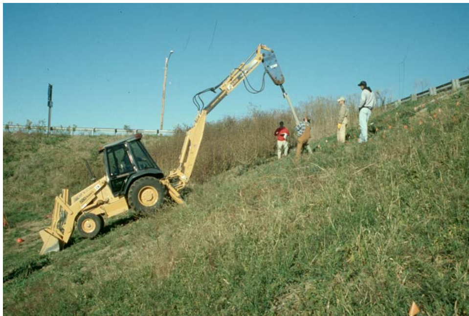
Figure 4. Backhoe-mounted hydraulic hammer use for initial installation attempts.
