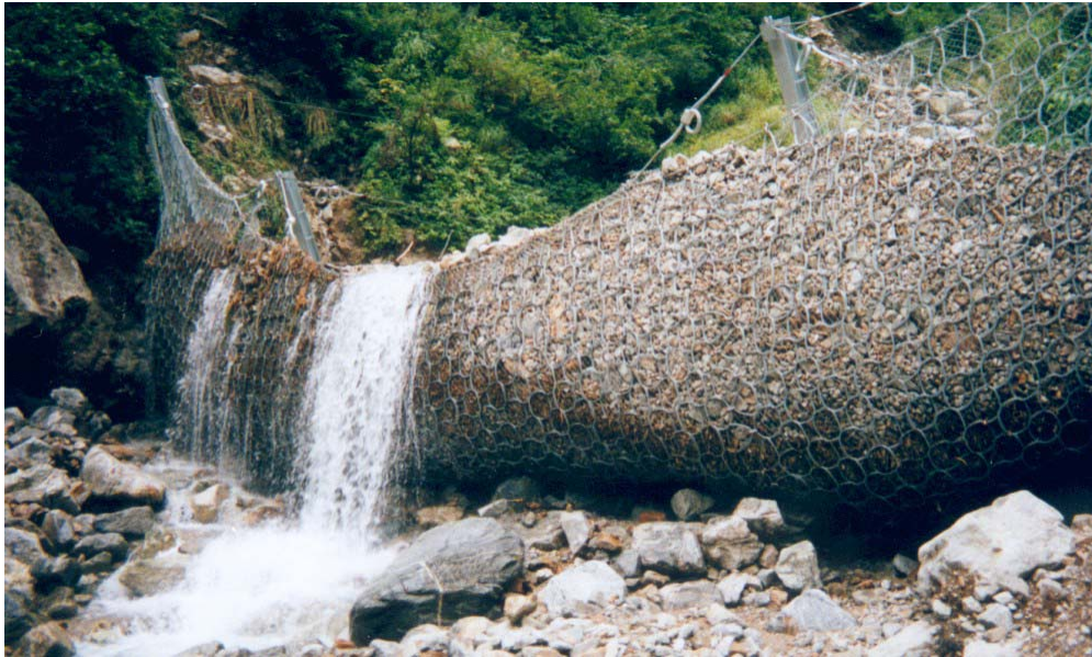
Figure 1 - Aobandoni, Japan Debris Flow Impact. 5 meter tall barrier.
