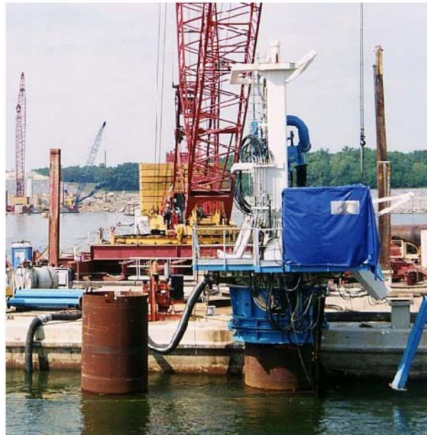
Figure 8: WIRTH Pile-Top Drill
