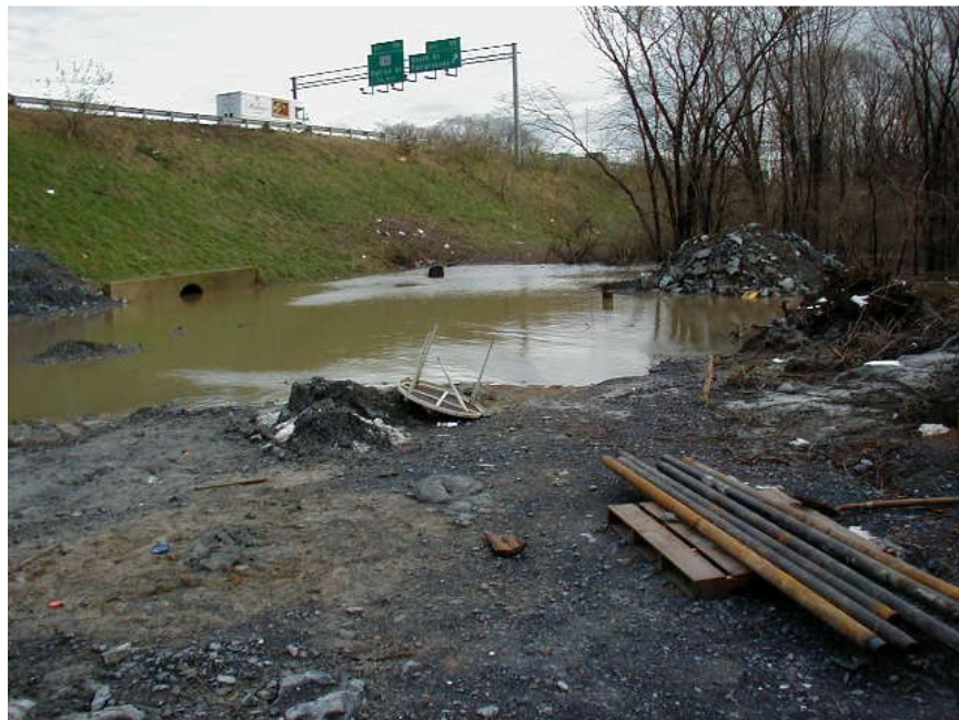
View of south pond area during heavy storm event. Note that the grouting has arrested the development of sinks for the time being.
