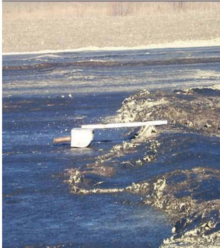
Figure 1. Vertical heaves generated after a rainfall event is the product of lime stabilization of a sulfate-rich subgrade.
