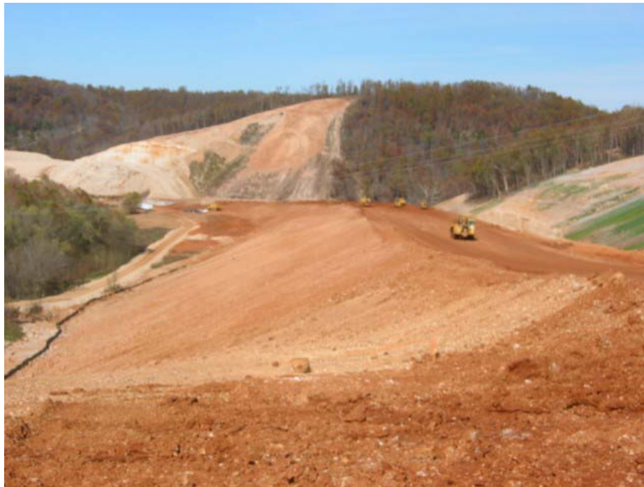
Figure 4: View of Completed 70-high Embankment at 2.5:1
