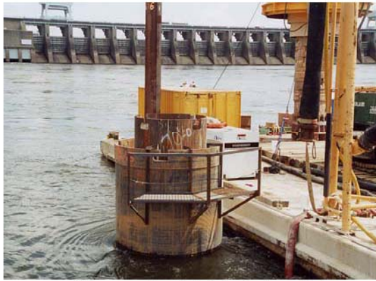
Figure 6: Shield Casing Setup
