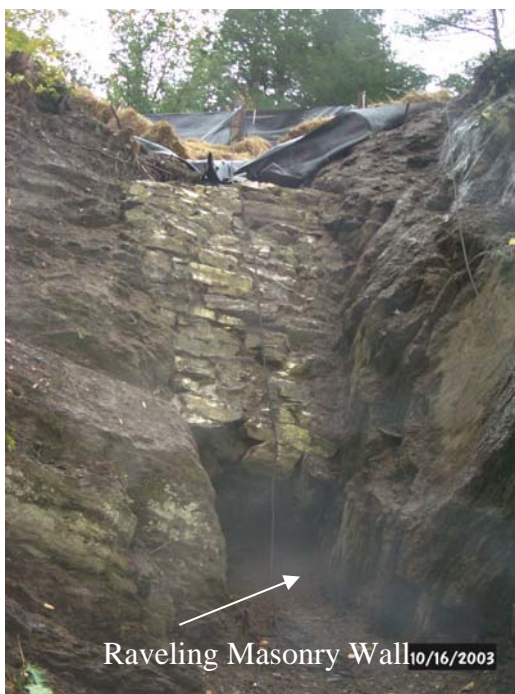
Figure 7: Masonry wall below washout.
