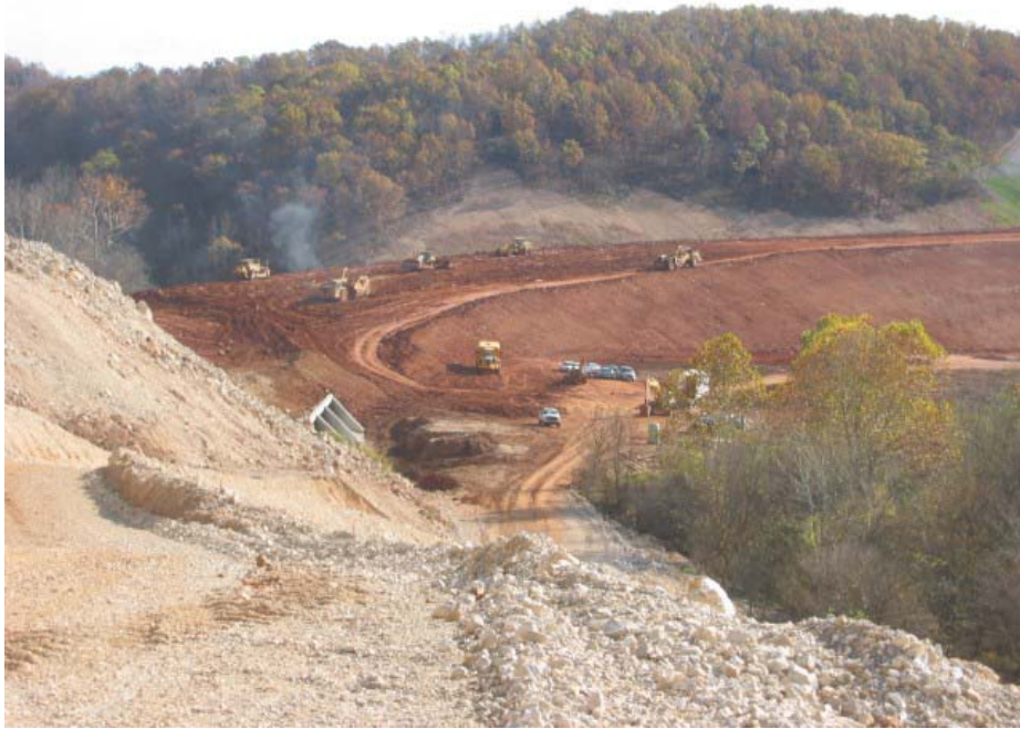
Figure 3: Embankment Construction over Landfill
