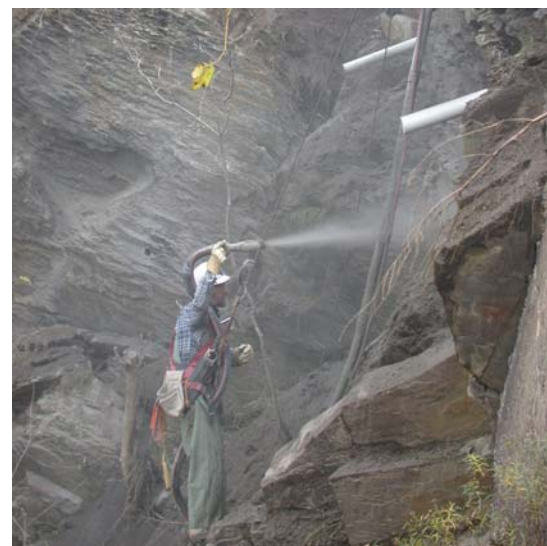
Figure 5: Shotcrete being applied while on rappel.
