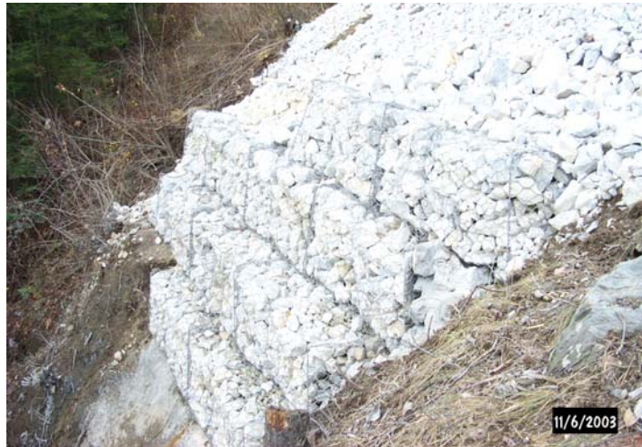
Figure 10: Completed Gabion wall
