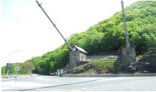
Figure 4: Existing eastern cable anchorages at the base of Anthony's Nose Mountain.
