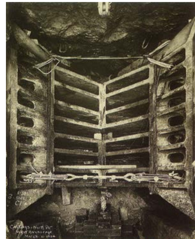
Figure 6: 1924 photograph showing end bearing castings in the anchorage tunnel. From "Bear Mountain Bridge – The History," by the New York State Bridge Authority.
