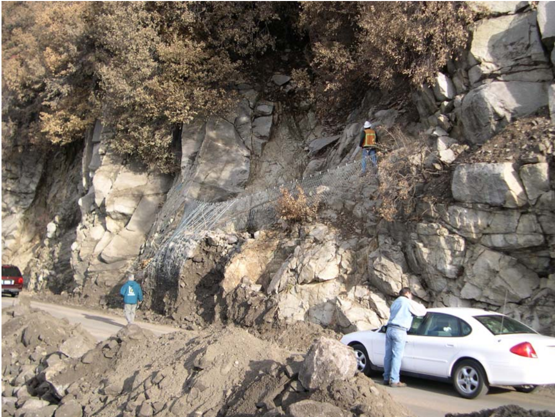
Figure 7 – Debris in and Around Suspended Tecco Mesh Drape
