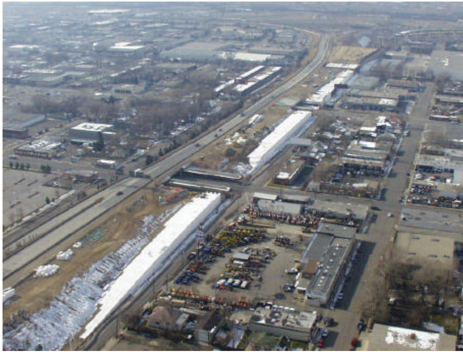
Figure 3. Geofoam Along Widening of Interstate 80
