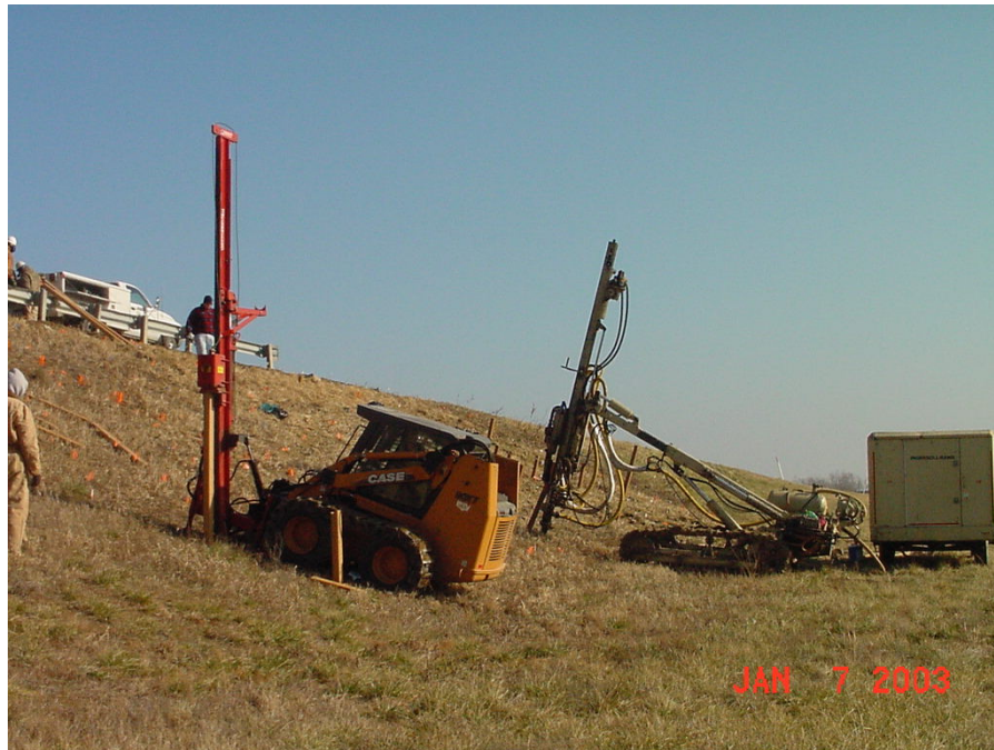
Figure 5. Pneumatic hammer drill (background) and drop-weight hammer rigs (foreground) successfully used to install reinforcing members at field test sites
