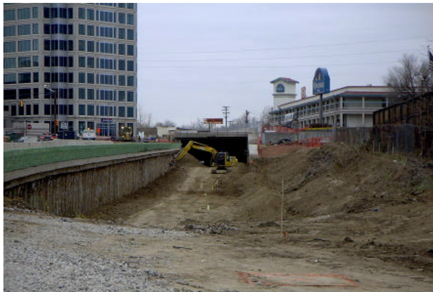
Figure 12: Adjacent Structure Next to Drilled Shaft Retaining Walls
