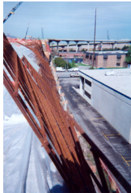
Figure 4. Wall SS-01 over Lime Cement Column area. Note, proximity of Nearby Building
