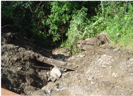
Figure 2: Washout of timber cribbing above mortared masonry wall. (View from road level)
