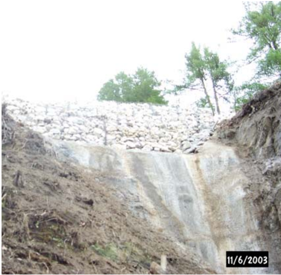
Figure 11: Completed repairs to mortared masonry wall below slide area.
