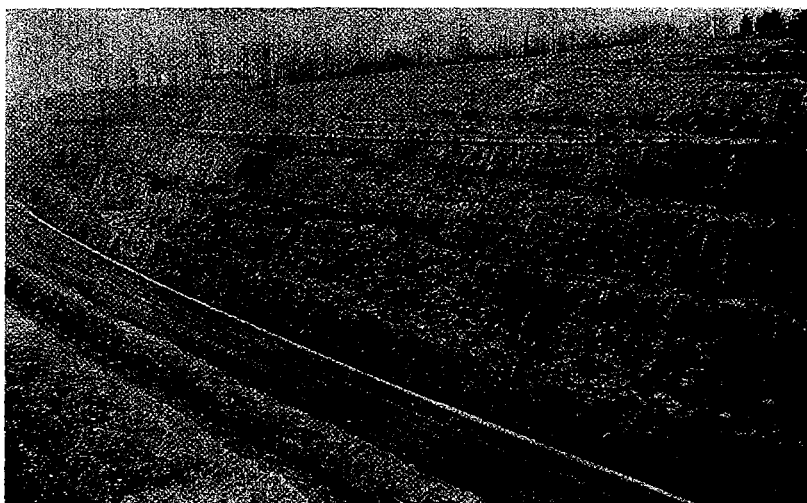
Figure 12. Same cut on I-64 looking west. A prominent 2 to 3 foot thick limestone layer, approximately 40 feet from the top, is visible.
