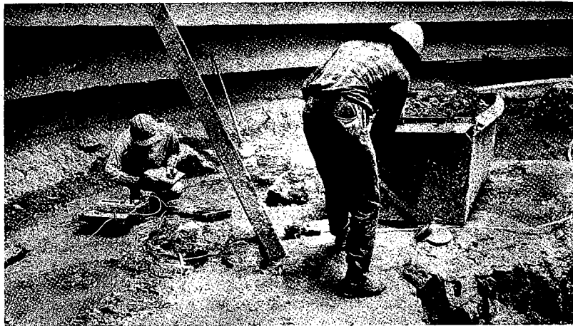
Figure 20. Plotting refraction seismic data of bedrock soundings (above), and conducting refraction seismic soundings (below) at bottom of Rouge River bridge caisson.
