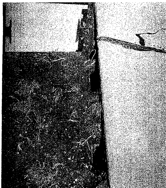
Figure 6. First stage blowhole on a crushed stone subbase, U.S. 41, Kentland Indiana
