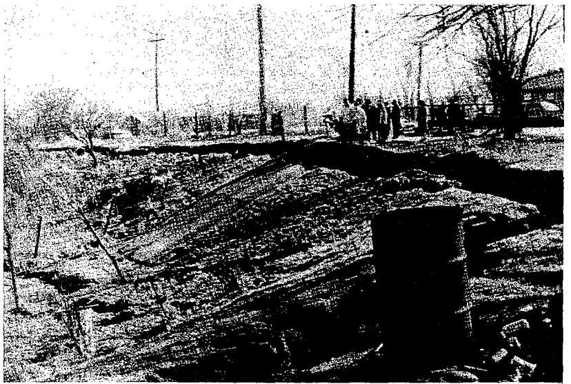
Figure 4. Tension cracks around outside of cave-in
