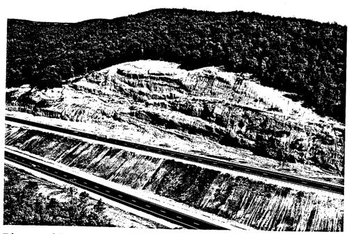
Figure 25. The median cut section of the big cut interval was flattened and relocated to reduce rockfall events in the lower east bound lanes of I-40 (photo by George Hornal).
