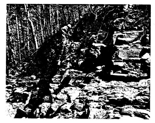
Figure 6. Hand scaling along I-40 in Cocke County helps to remove possible rockfall debris.
