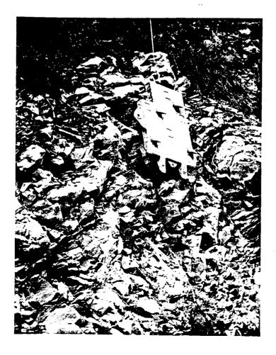
Figure 7. This 4'x5' (1.2x1.5m) metal plate was used in scaling rock slopes.
