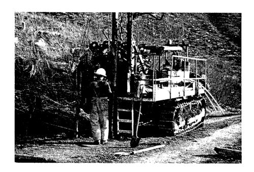
Figure 2. Steel Tracked Caterpillar Type Mounted Drill
