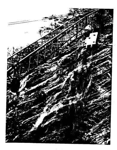
Figure 8. Scaling rock slopes along I-40 in Cocke County amounted to "sanding" the rock face of loose debris.
