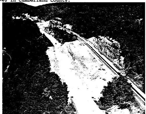
Figure 21. The section of I-40 in Cumberland County showing the precipitious rock cuts as the remedial project was initiated (photo by George Hornal).
