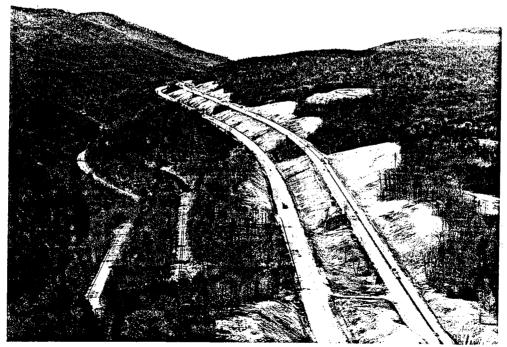
Figure 23. A completed section of I-40 in Cumberland County showing the results of the slope flattening concept (photo by George Hornal).
