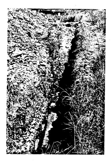
FIGURE 3. View looking east along trench T1 in borrow ditch on south side of U.S. Highway 14. Length of trench is 27 ft. Height of north wall is 6 ft. Water depth in trench is as much as 2 in.
