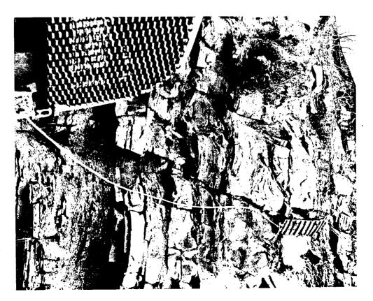
Figure 17. Dozer tracks were pulled back and forth across rock slopes as a method or scaling.
