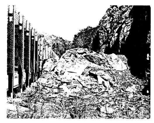
Figure 12. Rockfall catchment fences have proven to be beneficial as constructed along I-40 in Cocke County.
