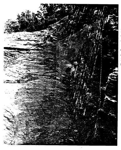
Figure 11. A draped catchment and rock control fence was constructed across wedge failure "V" shaped scars.
