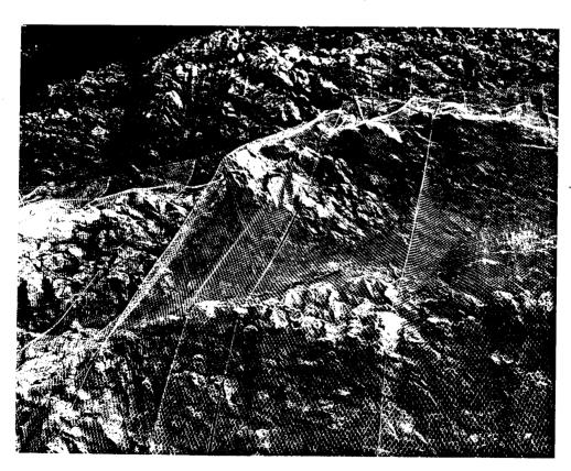
Figure 9. Draped wire meshing was used extensively along sections of I-40 in Cocke County.
