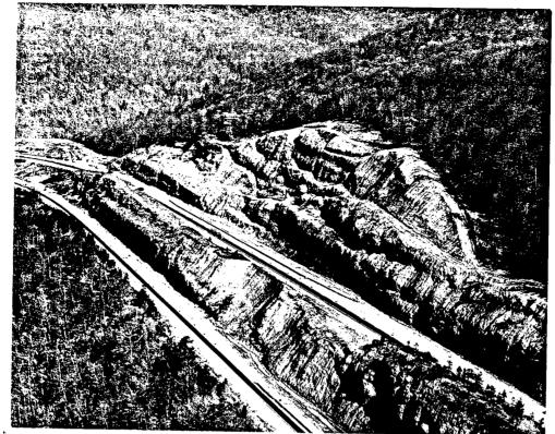
Figure 24. This photo shows the large 300' high (91m.) cut prior to slope flattening of the median. Scaling of the high slope has been completed (photo by George Hornal).
