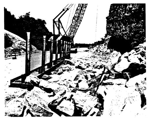
Figure 18. Portable catchment fences were used during the scaling project.
