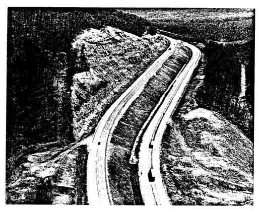
Figure 26. The upper west bound lanes of I-40, Cumberland County were shifted 40 to 60 feet (12 to 18 m.) away from the high cut slope, providing an adequate catchment area (photo by George Hornal).
