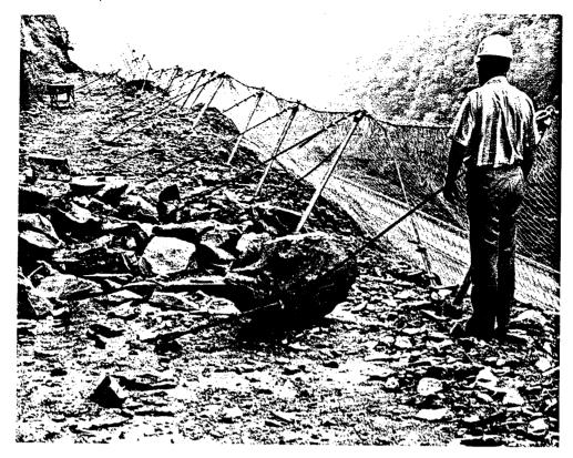
Figure 10. Rockfall control fences were constructed along the outer edge of in-slope benches
