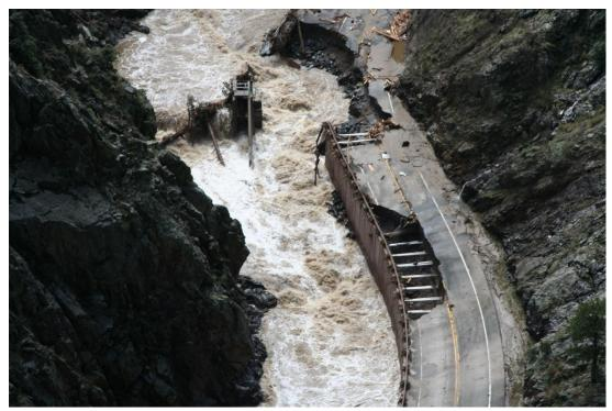
Figure 11. Destroyed Section of Highway Between Walls at Dille Dam.
