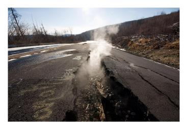
Figure 11 Subsidence Feature with Steam from Underground Mine Fire Old RT61 in Centralia, PA
