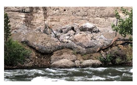
Figure 2. Photograph of from across the river showing the containment of essentially all material that was to be pinned to the slope by the temporary flexible fence.
