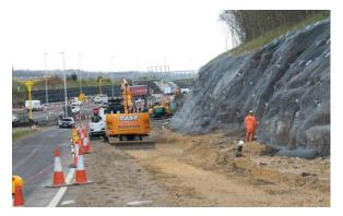
Figure 19 Mitigation of Cut Instability Using Mesh and Bolts, Newcastle, UK
