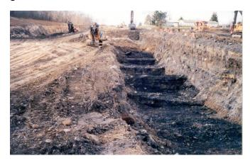
Figure 26 Over-Excavation of Mine Workings
