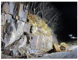
Figure 12. Rock scaling consisting of pry-bar, picks, and/or shovels. Where large rock blocks require removal, several different techniques can be used including inflatable air bags, hydraulic splitters, and winching as well as mechanical methods using conventional excavation equipment.
