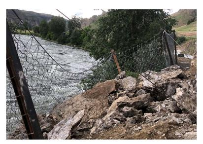
Figure 3. Photograph of from across the river showing the containment of essentially all material that was to be pinned to the slope by the temporary flexible fence.
