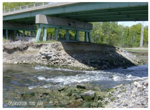
Figure 6. Failure of temporary post-breach stabilization.
