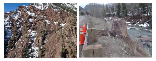
Figure 3: (a) source of MP 53.5 rockfall event (b) large boulder displaced at site. The boulder traveled across both lanes of SH 133 and came to rest above the neighboring creek.
