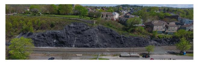
Figure 6. Photograph of sculpted shotcrete facing on a slope along a rail line in Hudson, NY. The project included over 300 cubic yards of shotcrete and rock bolts which would be a permanent solution to the issue of rock raveling into the track.
