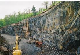
Figure 6 – Blasting and Rock Slope Excavation
