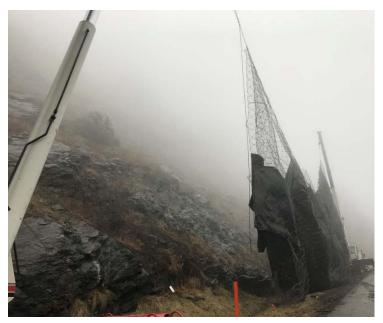
Figure 4. A temporary barrier hung from cranes on each end of scaling extents. System consists of various sizes of mesh to contain 100% of material.
