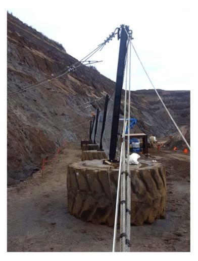
Figure 5. Photograph showing the above-grade footings for a semi-permanent rockfall which were constructed using recycled tires as form work for the concrete.
