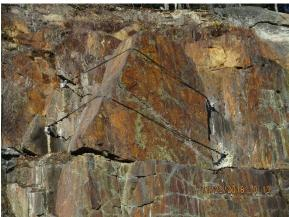
Figure 11 – Wire Mesh Netting and Wire Rope Cable Lashing in Areas 5 and 5A
