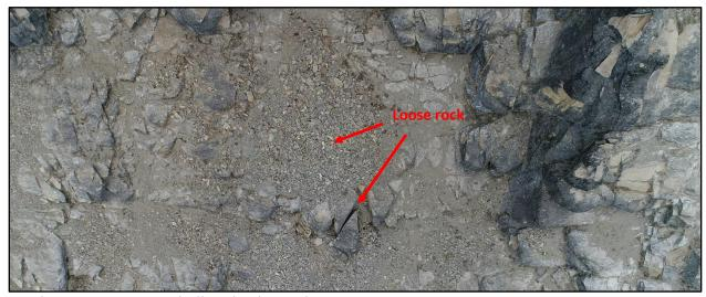
Figure 22: Loose rock directly above chute 3.
