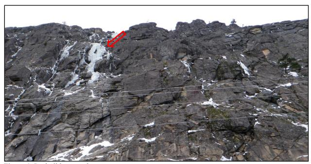
Figure 4: Ice build-up on slope.
