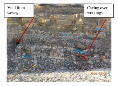
Figure 18 Example of Broken and Caved Rock and Void Exposed in Cut Above Mine Workings, Newcastle, UK
