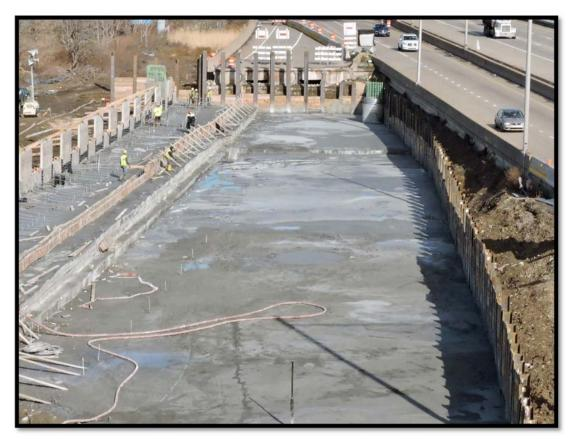
Figure 7: Compensating Fill Construction with Precast Facing Panels
