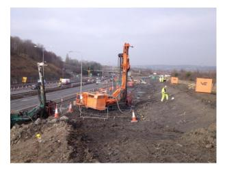
Figure 22 Grouting for Proposed Roadway Widening in UK
