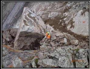
Figure 9: Estimate average block size and maximum block size one can expect on the slope. Blocks on left average about 2 ft diameter. Pyramidal block on right next to the geologist measures about 12 x 13 ft.
