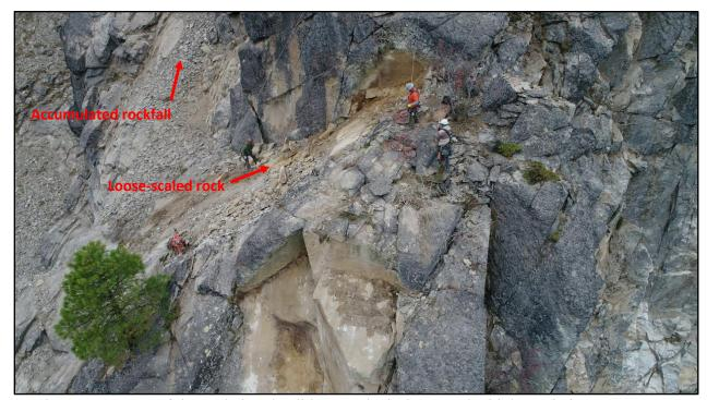
Figure 21: Many of the scaled rocks did not make it down to the highway below.
