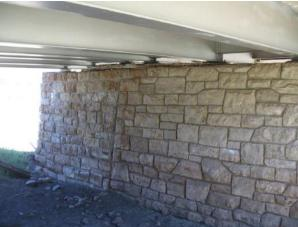
Figure 2 –Willow Valley Creek Bridge (left) and close up photo of bridge pier (right); note the near vertical joint near middle of photo separating the original bridge structure on the right from the 1964 widening on the left.
