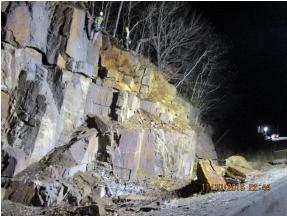
Figure 9 – Rock Slope Scaling at/near Area 9
