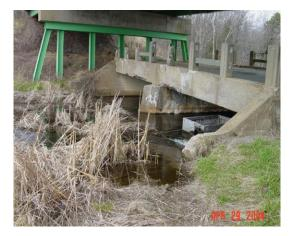
Figure 4. Suggested failure mode – the clogged spillway facing upstream in 1995 (a) and 2004 (b).
