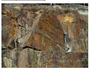
Figure 11. Wire rope cable lashing
