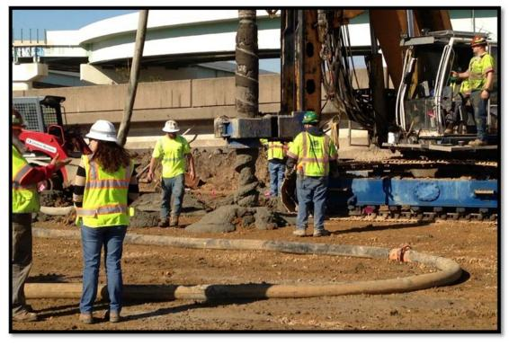
Figure 8: Column Supported Embankment Drilling Operation
