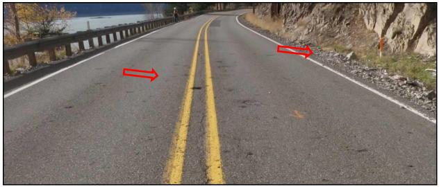
Figures 13: Rockfall in the ditch and pavement divots below the slope.
