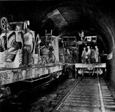
Figure 20 View of Rook Tunnel Repairs with View on Left of Liner Plates Covered with Mesh in Preparation for Shotcrete Placement and View on Right Showing Shotcrete Placement (Railway Age, 1942)
