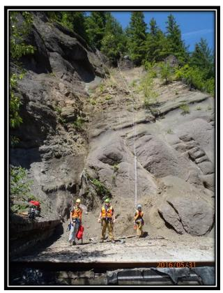
Figure 10: In the left photo, the investigator is assessing the slope, checking for rockfall conditions and the adequacy of the catchment ditch along the railway. In the right photo, the climbers are standing at the base of a large rock chute which is source of major rockfall.
