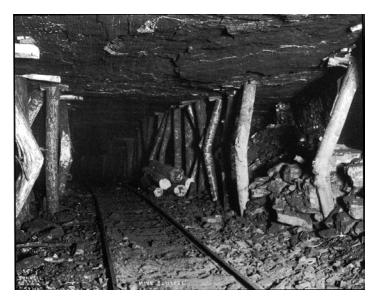
Figure 7 Squeeze (Creep) at Mine Level in Anthracite Region of Pennsylvania Bartoletti, 1996
