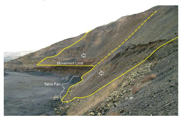
Figure 8 – Landslide Debris, Talus Fan, and Rockfall in Quarry Floor (March 22, 2018)
