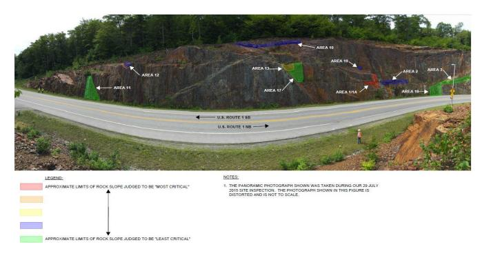
Figure 8-Rock Slope Remediation Area (Sheet 2 of 2). This view shows the southern portion of the rock
