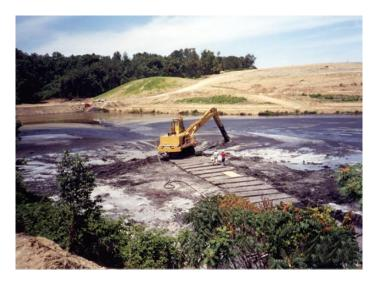
Figure 13 Constructing a Road Over a Slurry Pond in Pennsylvania
