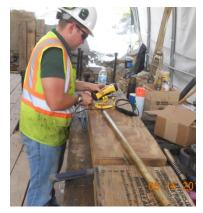
At predetermined intervals the boring is surveyed using the multishot survey tool. The photograph at left shows our engineer downloading the survey data from the multishot tool. He then plots the "as drilled" coordinates against the borehole plan coordinates to assess what steering maneuvers are needed. Surveying the borehole as it advances is important as the drill
