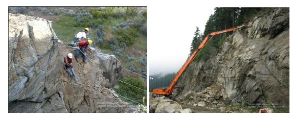
Figure 1: Mechanical Scaling and Hand Scaling. (Photos Courtesy of the Transportation Research Board)
