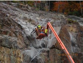
Figure 10 – Rock Dowel Drilling with Wagon Drill (left) and Manlift (right)
