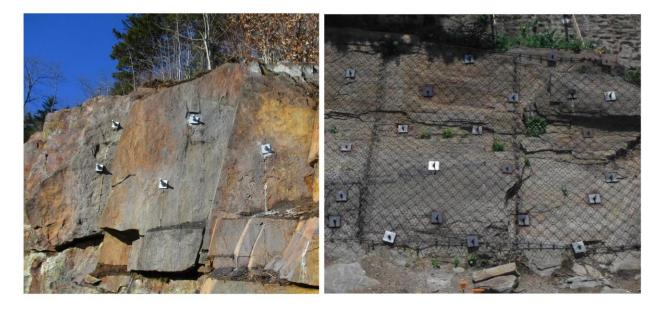
Figure 3. Photographs of rock dowels (left) and anchored mesh (right).
