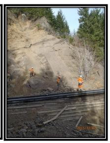
Figure 7: Example of width and height of slope. In this case the slope width measured at the toe is about 160 feet. The height measured from the brow to the toe is about 200 feet
