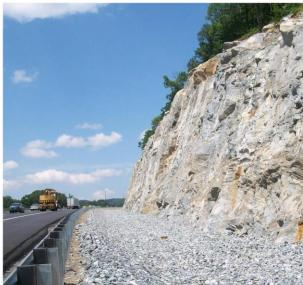
Figure 4. Photographs of rockfall barrier fencing (left) and a rockfall catchment ditch (right).
