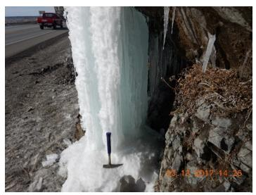
**Figure 5** – Partial ice column direct bearing near MP 113.2 NB on the Seward Highway (Photo by Scarptec, Inc.)
