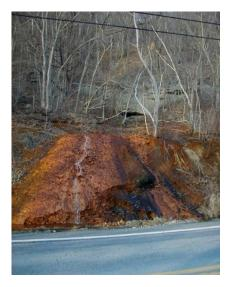
Figure 14 Acid Mine Drainage Flowing from Abandoned Workings in the Pittsburgh Coal Seam, RT 837 West of Elrama, PA. The Water Was Treated by Applying Limestone to the Slope.
