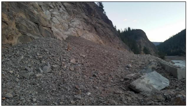
Figure 19: Scaling debris captured along the highway before it was cleared.
