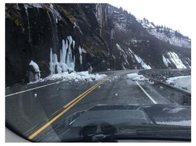
**Figure 7** – Direct icefall impact & shatter at MP 13.9 Richardson Highway. Slab partially rotated outward during fall from overhung slope on 13 December 2017. Photo courtesy of AKDOT&PF.
