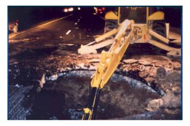
Figure 3 Over-Excavation of Sinkhole on I-70 in Ohio March 5, 1995
