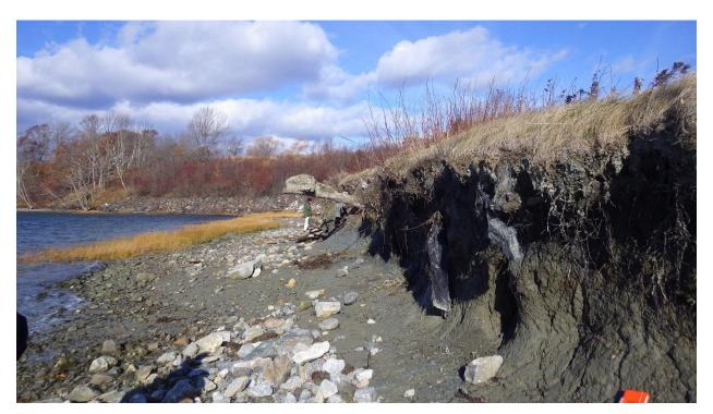
Figure 10: Photo of eroded 1996 landslide toe (taken 11/20/17, looking northwest), which has retreated to the rip-rap barrier that was installed within the toe during remediation. A tree that was swept up in the landslide is also visible in the bank, as well as rip-rap armor that extends beyond the landslide area in the distance. Photo: Lindsay Spigel.
