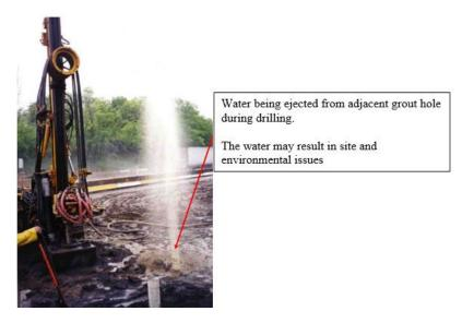
Figure 15 Water Being Ejected During Drilling into Flooded Mine Workings
