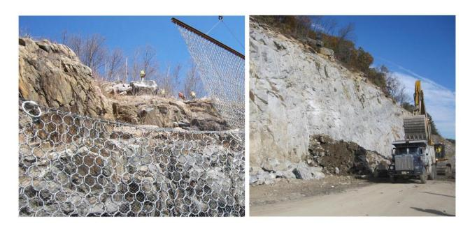
Figure 2. Photographs of rock scaling (left) and a trim-blasted slope (right).
