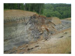
Figure 17 Close-Up of Slope Failure
