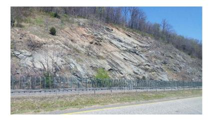
Figure 1: Structurally controlled failure (plane failure).
