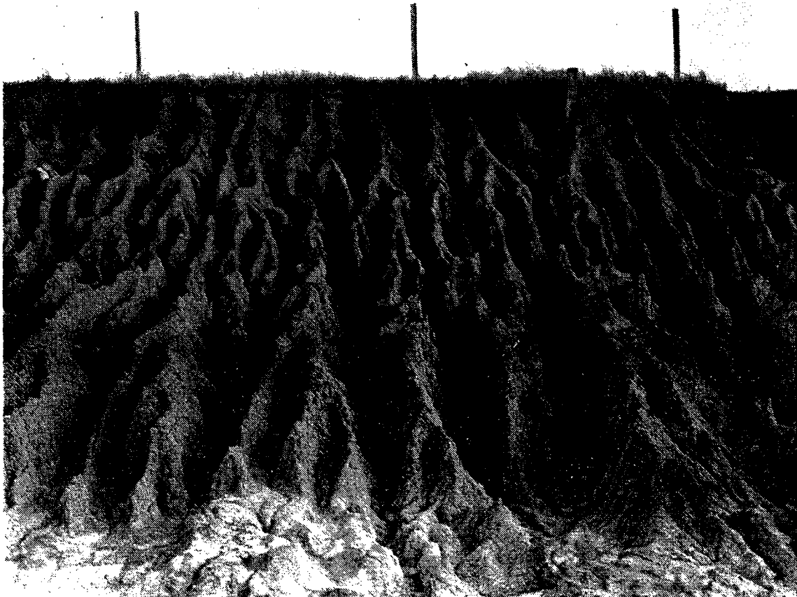
Figure 1. Loess on a 2:1 slope that was not properly sodded.
